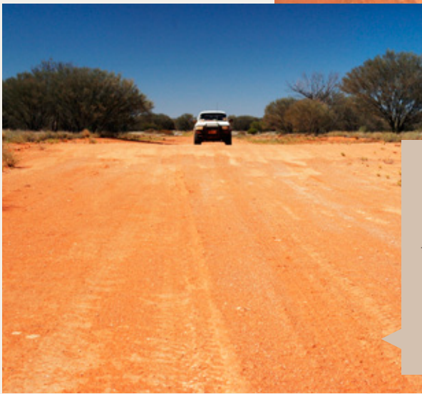
Photo 3b. A “track creek” with major sand deposition in the foreground and scouring in the background. Note the road is cut down and has windrows on both sides. Natural cross flow was from left to right before it was captured by the “road creek”. (Hugh Pringle EMU™)
