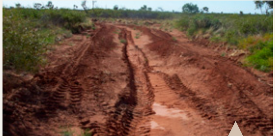
Figure 3 and Photo 5. V-shaped drains discouraged. (courtesy of the Northern Territory Government)
