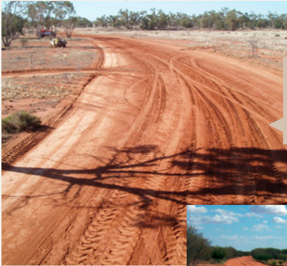
Photo 3b. A “track creek” with major sand deposition in the foreground and scouring in the background. Note the road is cut down and has windrows on both sides. Natural cross flow was from left to right before it was captured by the “road creek”. (Hugh Pringle EMU™)
